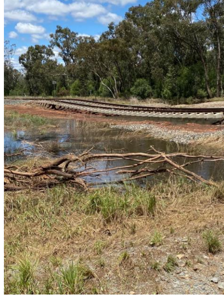
Plate C7.19 – Collapsed section of railway immediately to the east of Overland Road.
